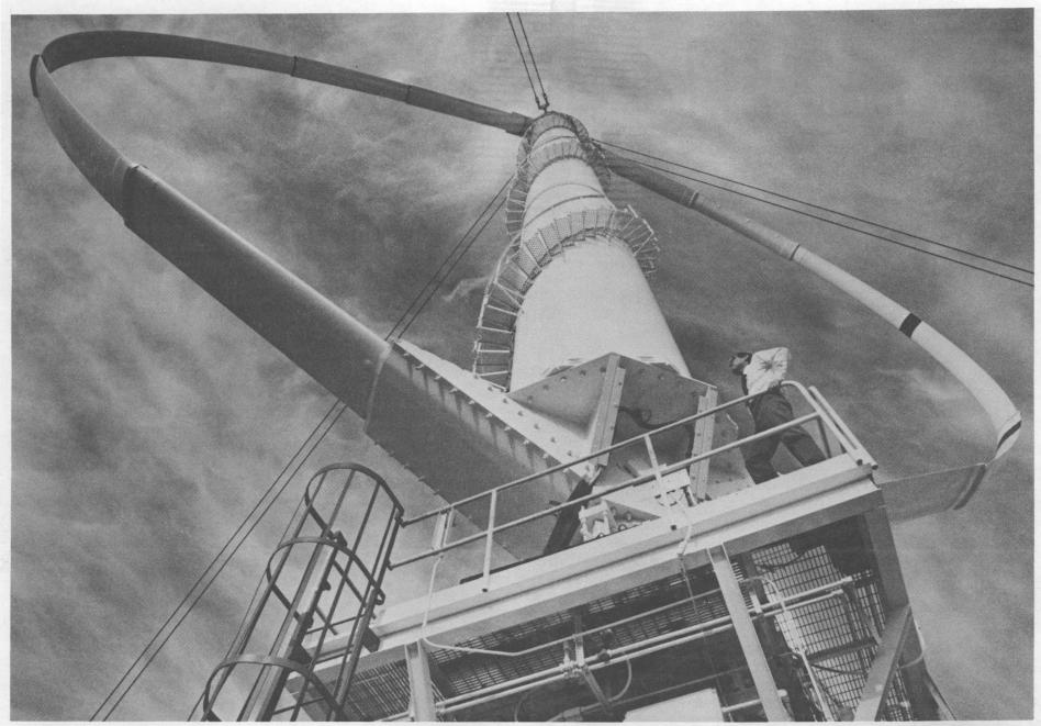
THE DOE/SANDIA VAWT (Vertical Axis Wind Turbine) Test Bed was dedicated last week in Bushland, Tex. Here, test engineer Bill Stephenson (6225) gazes up the windmill's 10-ft.-diam. vertical axis to the top of the 165-ft.-tall structure. The VAWT's two large, bowed aluminum blades — each spanning 183 feet — swing out from the column's axis; at their widest point, they are 110 feet (34 metres) apart. More information on Page Nine.
